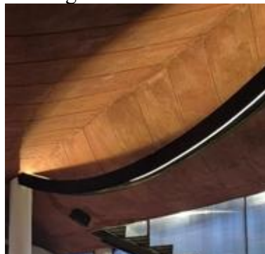
Figure 7. Lighting in the Visitor Area
