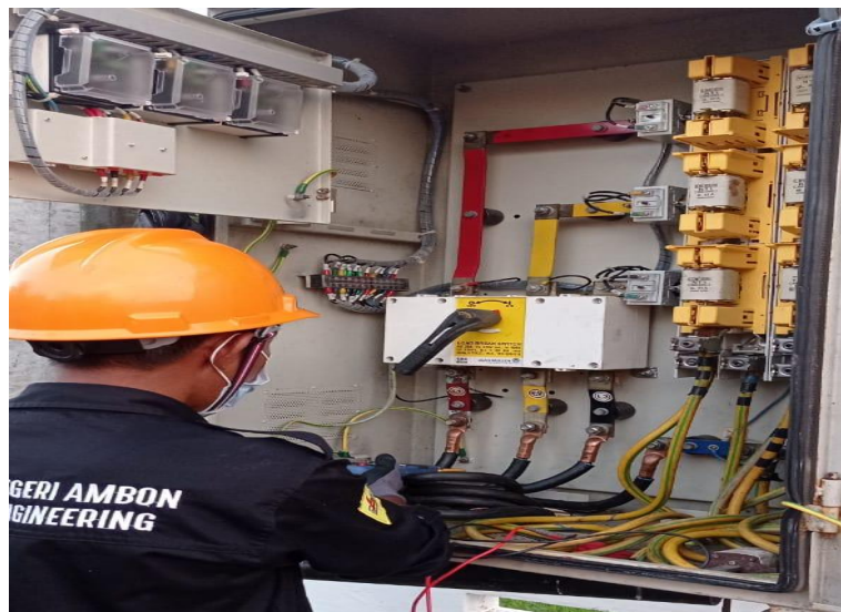
Figure 1 Manual Transformer Load Measurement
