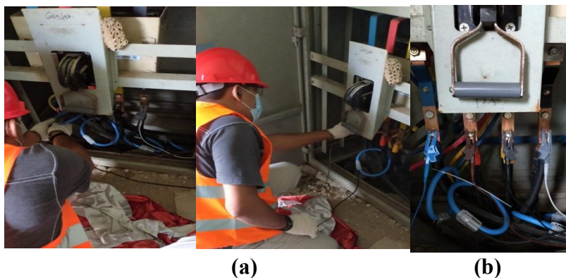
Figure 3. (a) Installation of clamp and jumper (b) Clamp and jumper attached to phase, neutral and ground wires
