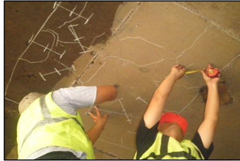
Figure 3. Distribution of crack patterns
