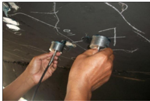
Image Crack depth check before injection.
