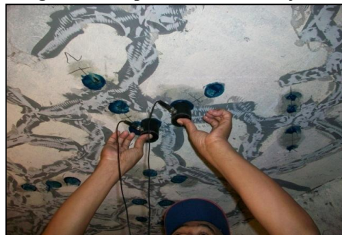
Figure Inspection of crack depth after injection
